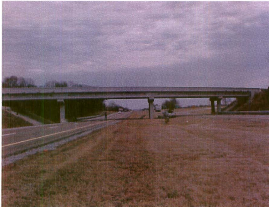
ELEVATION UNDER BRIDGE, DIRECTION OF ROUTE
